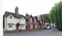
The prominence of tiled, gabled roofs.
