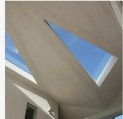
Sussex House by Wilkinson King. Triangular rooflights.
