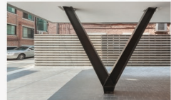
Nonhym Limelight Music Consulting by Dia Architecture. Exposed steel columns.
